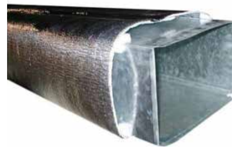
Installing insulation on HVAC ducts
